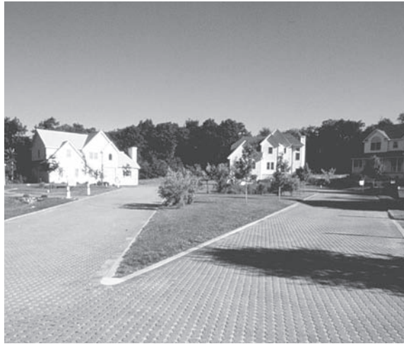
Figure 28. Besides expected decreases in stormwater, runoff monitored from permeable interlocking concrete pavement projects such as Glen Brook Green Subdivision, Waterford, Connecticut in the Jordan Cove Watershed demonstrate substantial reductions of pollutants compared to those from conventional pavements.
