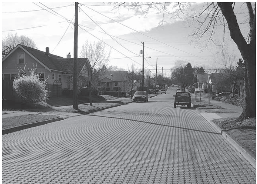
Figure 11. Portland, Oregon renovated streets with about 20,000 sf (2,000 m 2 ) of permeable interlocking concrete pavement after water and sewer line repairs in an older neighborhood. The city incorporated modeling to evaluate this pavement. The pavement decreased combined sewer overflows to the waste treatment plant and discharges to into the Willamette River.
