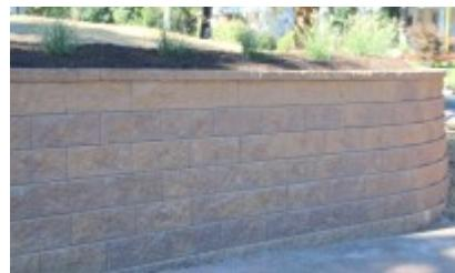
Set all wallstones with knobs protruding down, so that one knob will drop into each core of the wallstone below establishing a bond. Pull the wallstones forward and center on the bond of the two wallstones below. All full-on bond wallstones are set in this way. Corners and cutting a wallstone for adjustment are discussed in the corner section of this handbook titled: Sigma 6-Inch Corner.
