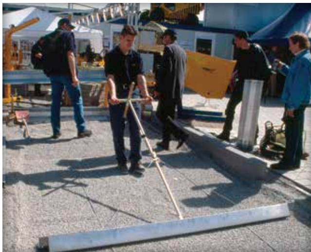
Figure 24. Manually screeding the No. 8 stone setting bed.
