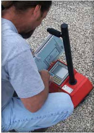
Figure 23. Density testing with a nuclear gauge in backscatter mode can help assess consistent density of the ASTM No. 57 base layer.
