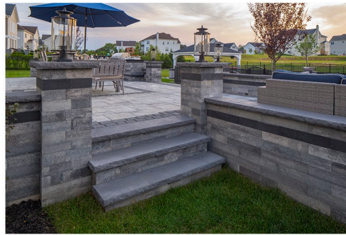
Raised Patio Construction
