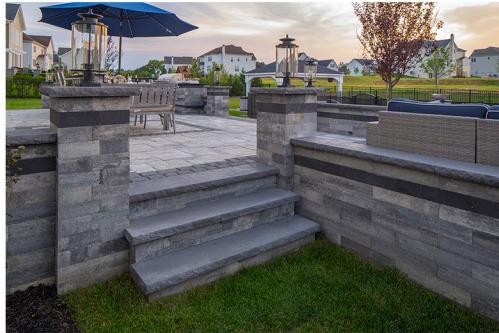
Raised Patio Construction
