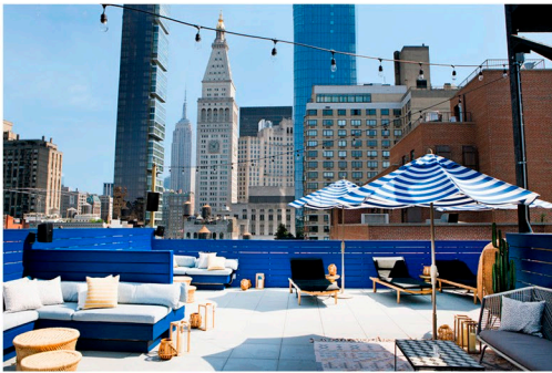
Rooftop Paver Pedestal Installation
