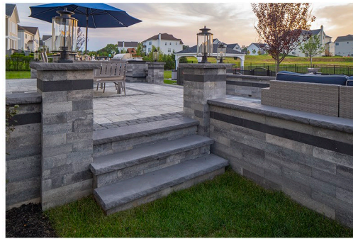
Raised Patio Construction
