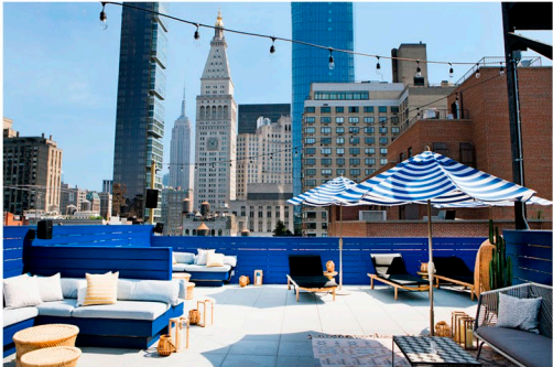
Rooftop Paver Pedestal Installation
