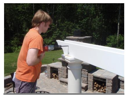
HOLD LINTELS IN PLACE AGAINST THE POST CORE WITH A CLAMP. PLACE A LEVEL ACROSS THE TOP OF BOTH LINTELS (PARALLEL AND PERPINDICULAR) TO INSURE THEY ARE LEVEL. DRILL THRU EACH LINTEL AND THE FIBERGLASS POST CORE IN A SINGLE PASS.
