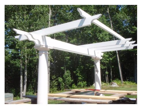
Set then and level the leftmost and rightmost rafters first. Then set the backmost and front most purlin. Double check that both the rafters and the purlins are level. Begin installing the remaining rafters and then install the remaining purlins.
