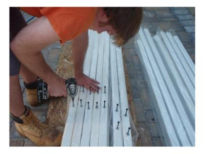
Predrill and set the screws into the rafters on the ground first. Maximum cantilever is 3 feet from the back tip of the rafter to the back beam (lintel) and five feet from the back beam to the front tip of the rafter.
